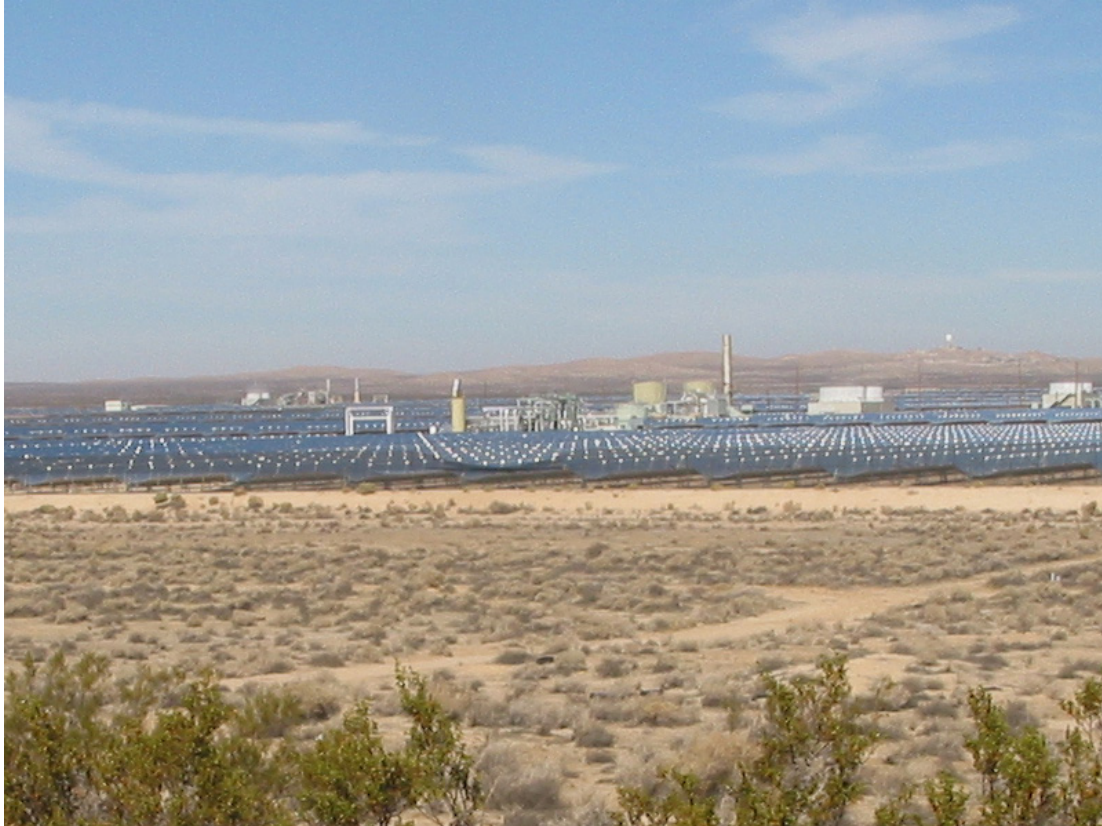
Figure 6. Geometric pattern of reflected light on SEGS III-VII parabolic trough facility (3.9 km 2 [970 acres]). Photo taken October 29, 2008, 1:30 PM, direction of view not available, solar azimuth of 179° and solar elevation of 41°.
