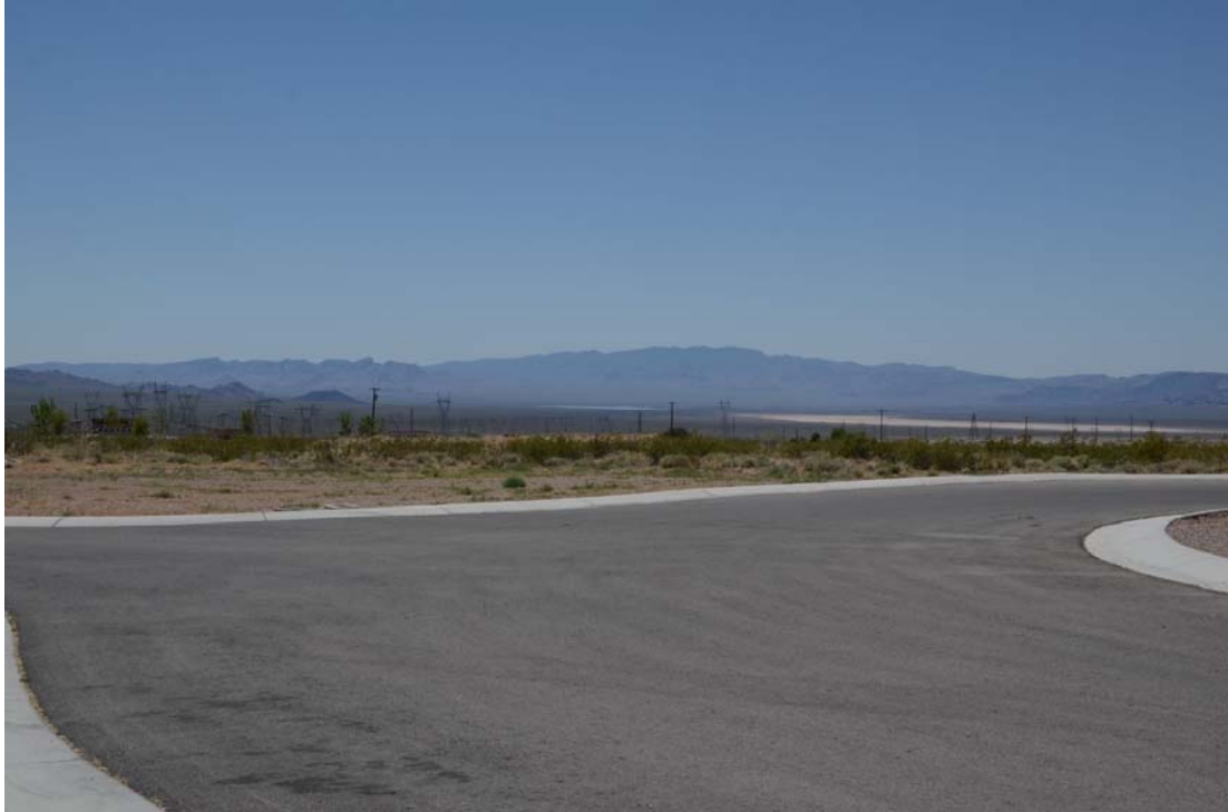
Figure 3. Nevada Solar One parabolic trough facility (1.6 km 2 [400 acres]), as seen from a distance of approximately 23 km (14 mi). The Nevada Solar One facility is the narrow white band at the center of the photo. Photo taken May 5, 2011, 12:14 PM, looking southwest, solar azimuth of 131° and solar elevation of 63°.
