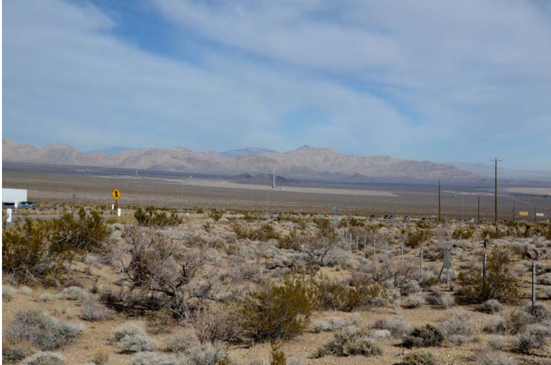
Figure 1. Partially completed Ivanpah power tower facility, as seen from a distance of 6.8 km (4.2 mi) from the Unit 1 tower (at center). The cleared area at center is approximately 2 km (1.25 mi) across, and covers 3.66 km 2 (900 acres). Cleared areas and two additional towers are visible in the distance at left. The facility eventually will cover 14 km 2 (3,400 acres). Photo taken January 20, 2012, 10:14 AM, looking northwest, solar azimuth of 139° and solar elevation of 23°.
