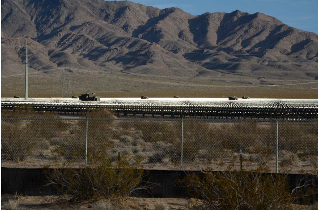
Figure 7. Geometric pattern of reflected light on Silver State North PV facility (2.4 km 2 [600 acres]). Photo taken January 26, 2012, 4:06 PM, looking south-southeast, solar azimuth of 228° and solar elevation of 19°.
