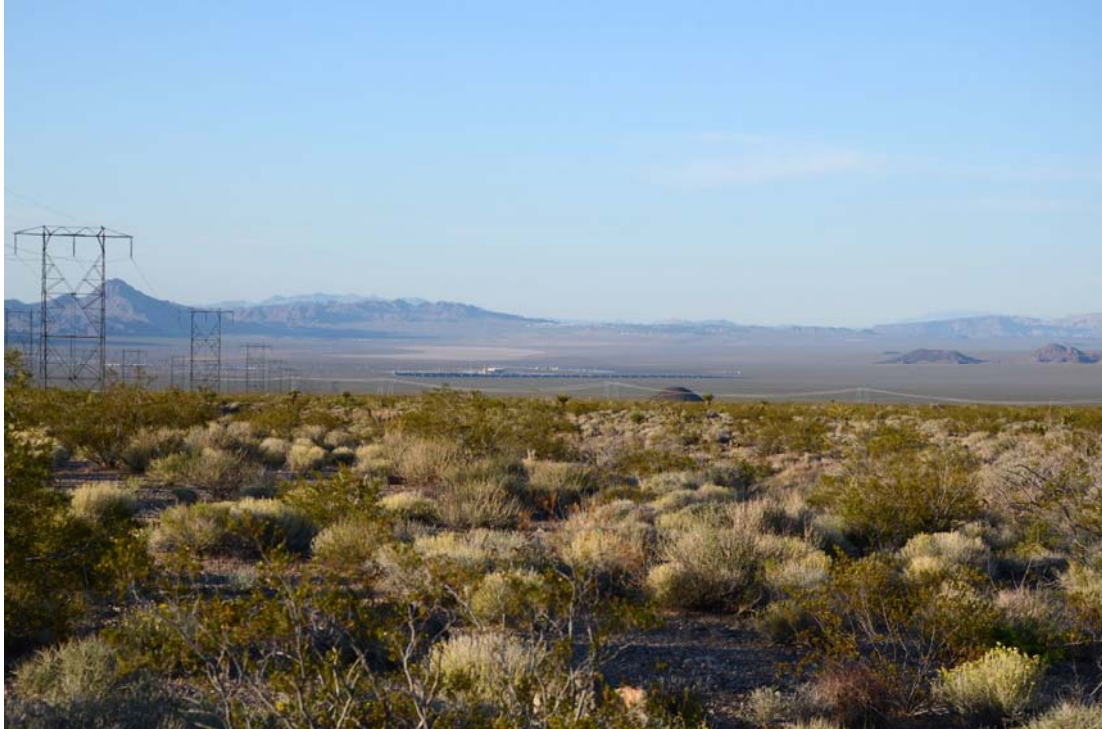
Figure 2. Copper Mountain thin-film PV facility (1.5 km 2 [380 acres]), as seen from a distance of approximately 13 km (8 mi). The facility is the black line across the center of the photograph; lighter objects immediately above the facility are components of a natural gas power plant. Photo taken May 2, 2011, 6:39 PM, looking northeast, solar azimuth of 275° and solar elevation of 21°.
