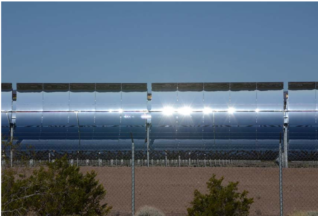
Figure 5. Glare sources on Nevada Solar One parabolic trough facility. The glare sources appear to be associated with the heat transfer fluid tubes and/or associated components attached to the tubes. Photo taken May 5, 2011, 8:42 AM, looking southwest, solar azimuth of 86° and solar elevation of 23°.
