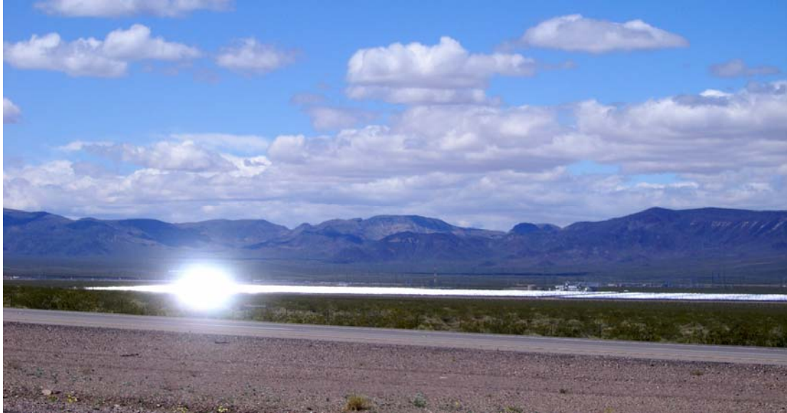
Figure 4. Glare spot on Nevada Solar One parabolic trough facility (1.6 km 2 [400 acres]), as seen from a slightly elevated viewpoint on U.S. 95. Photo taken April 21, 2010, 12:00 PM, looking southwest, solar azimuth of 131° and solar elevation of 57°.
