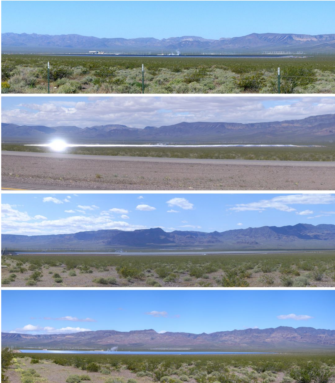
Figure 8. Color shifting of Nevada Solar One parabolic trough facility (1.6 km 2 [400 acres]) shown in the center of the four views. The color of the collector array may vary widely based on mirror position and the environmental features, such as clouds or sky that are reflected in the mirrors. Top photo: April 24, 2010, 8:04 AM, looking southwest, solar azimuth of 83° and solar elevation of 13°. Second photo: April 21, 2010, 12:00 PM, looking west-southwest, solar azimuth of 131° and solar elevation of 57°. Third photo: April 23, 2010, 2:32 PM, looking northwest, solar azimuth of 211° and solar elevation of 64°. Bottom photo: April 21, 2010, 9:49 AM, looking northwest, solar azimuth of 100° and solar elevation of 33°.
