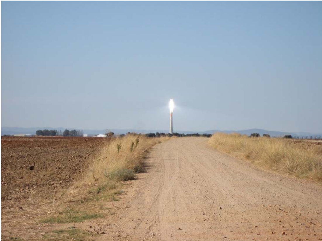
Figure 12. Torresol Gemasolar 19.9 MW Power Tower (1.85 km 2 [457 acres]). In addition to the intensely white receiver light, reflected light from dust particles in the air around the receiver is plainly visible. The light appears to stream both downward and upward from the receiver. The central tower is 140 m (459 ft) tall. Heliostats are visible at right. Photo taken September 23, 2011, 5:50 PM, looking north, solar azimuth of 246° and solar elevation of 28°.
