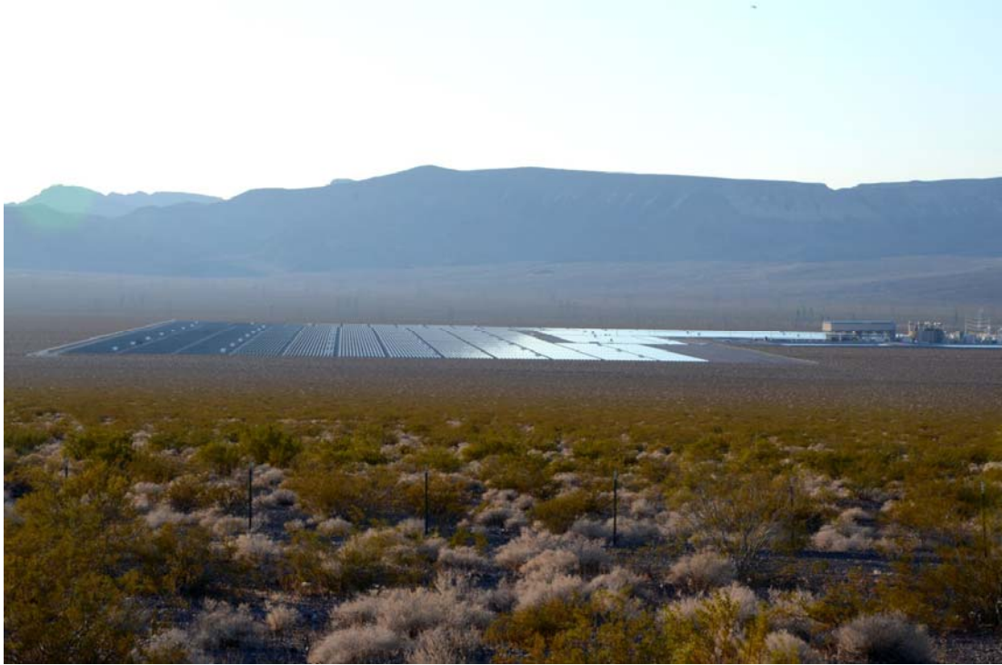
Figure 9. Color transition Copper Mountain thin-film PV facility (1.5 km 2 [380 acres]). Color changes from black to blue to white and back again as the facility is passed. Photo taken January 27, 2012, 4:13 PM, looking west, solar azimuth of 230° and solar elevation of 18°.
