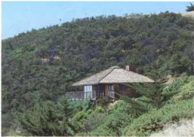
Top and middle — Attractive structures in the landscape, but also a high fire risk. Note the combustible roof, large glass windows, and overhanging deck in the middle photo.
