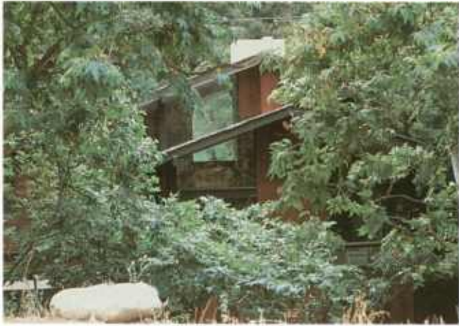
Top and middle — Attractive structures in the landscape, but also a high fire risk. Note the combustible roof, large glass windows, and overhanging deck in the middle photo.
