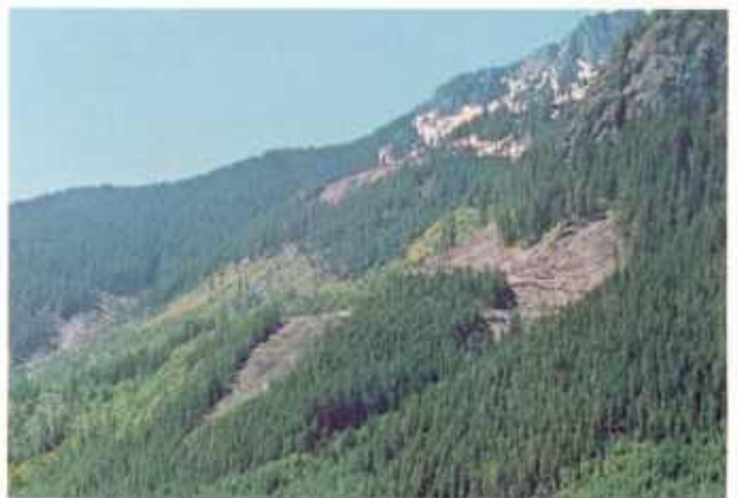
Roads and landings located and constructed to minimize cuts and fills.
