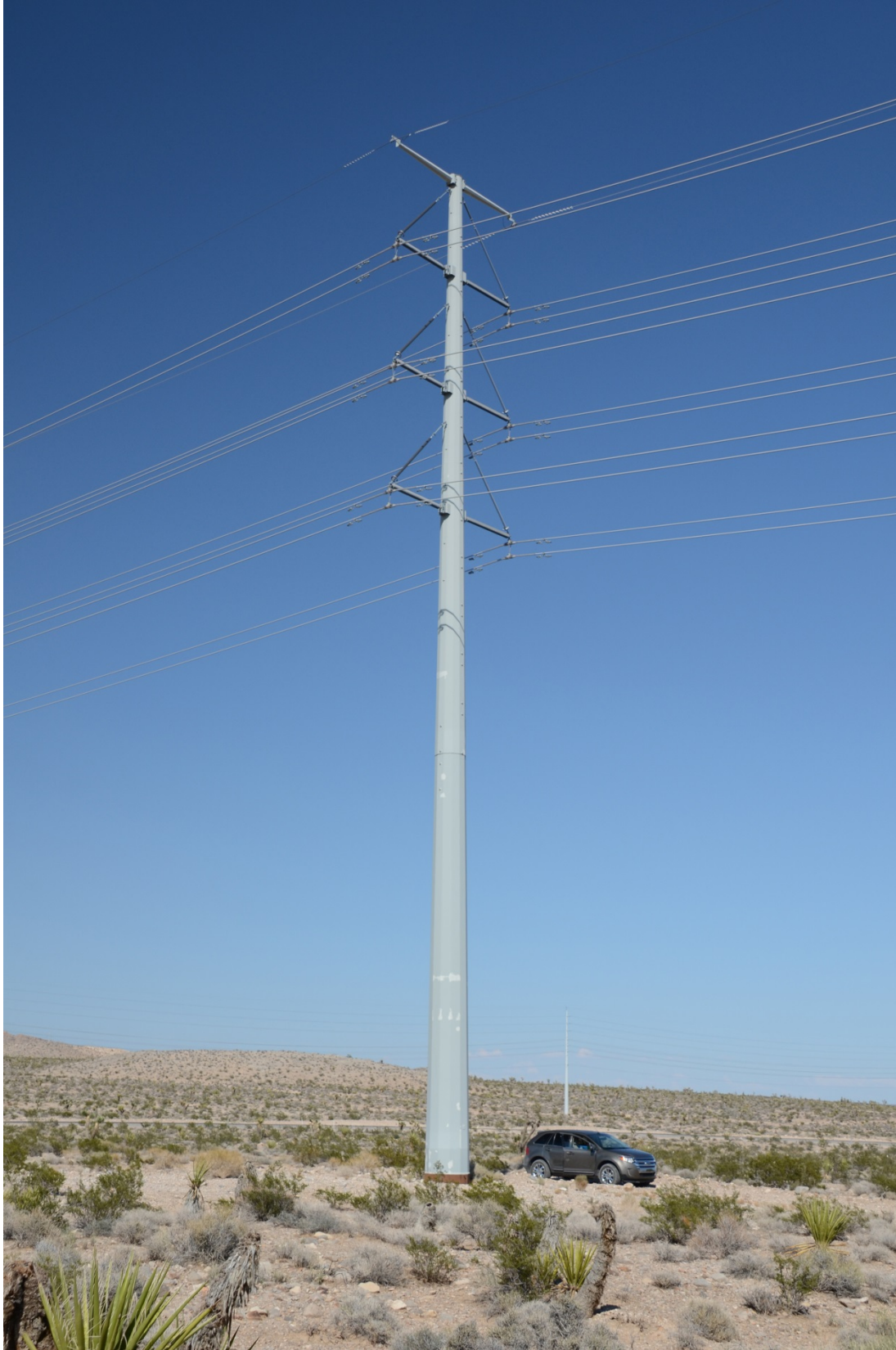
Figure 4. Bighorn 230-kV Monopole Transmission Tower
