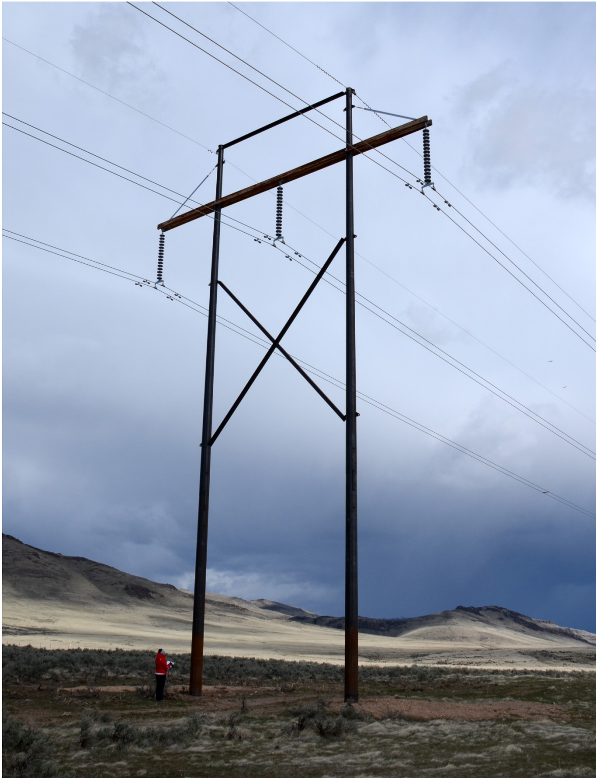
Figure 3. Mountain Home 230-kV H-frame Transmission Tower
