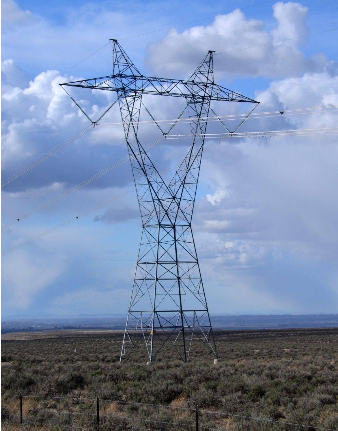
Figure 1. Midpoint-Summer Lake 500-kV Lattice Transmission Tower
