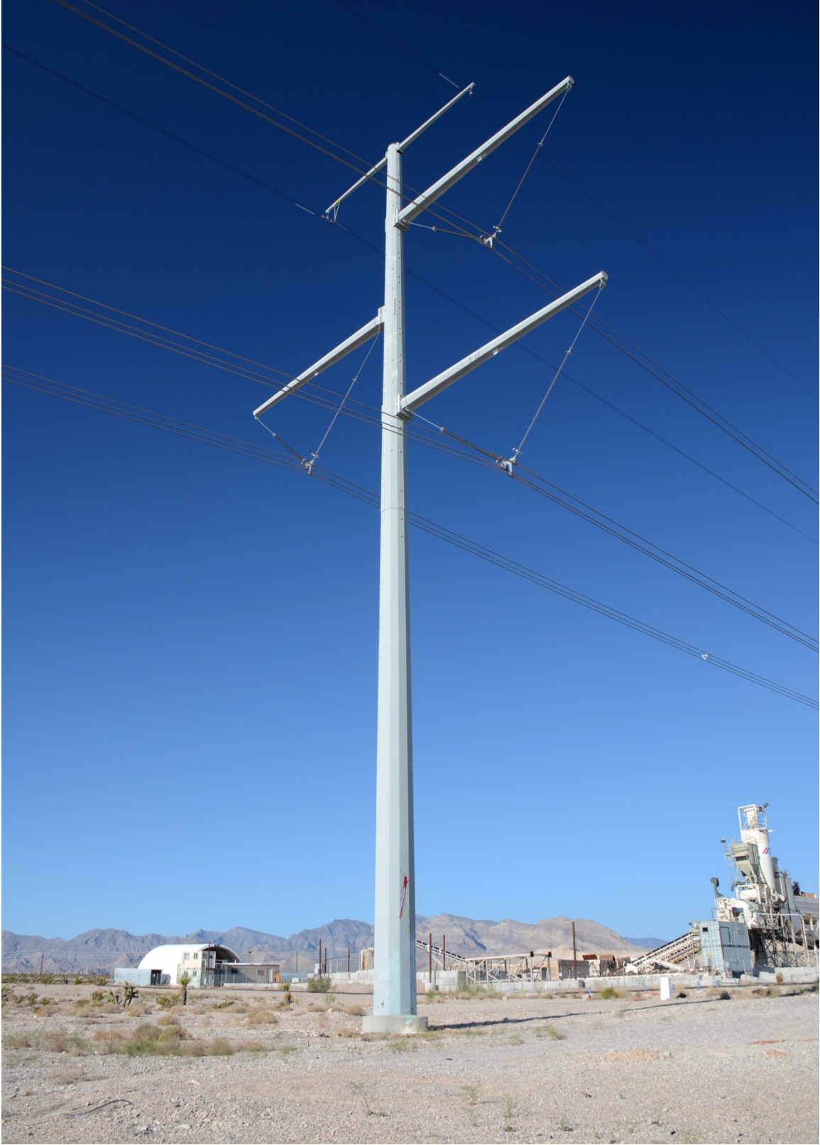
Figure 2. North Las Vegas 500-kV Monopole Transmission Tower
