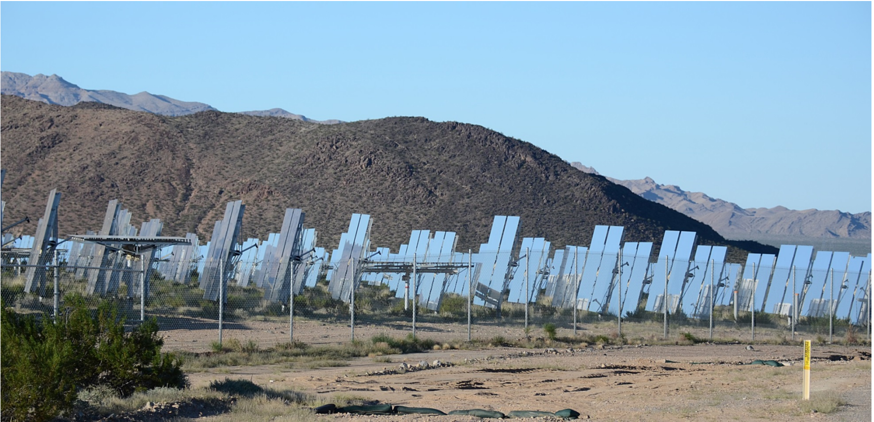
FIGURE 3.1-14 Close-Up View of ISEGS Heliostat Array
