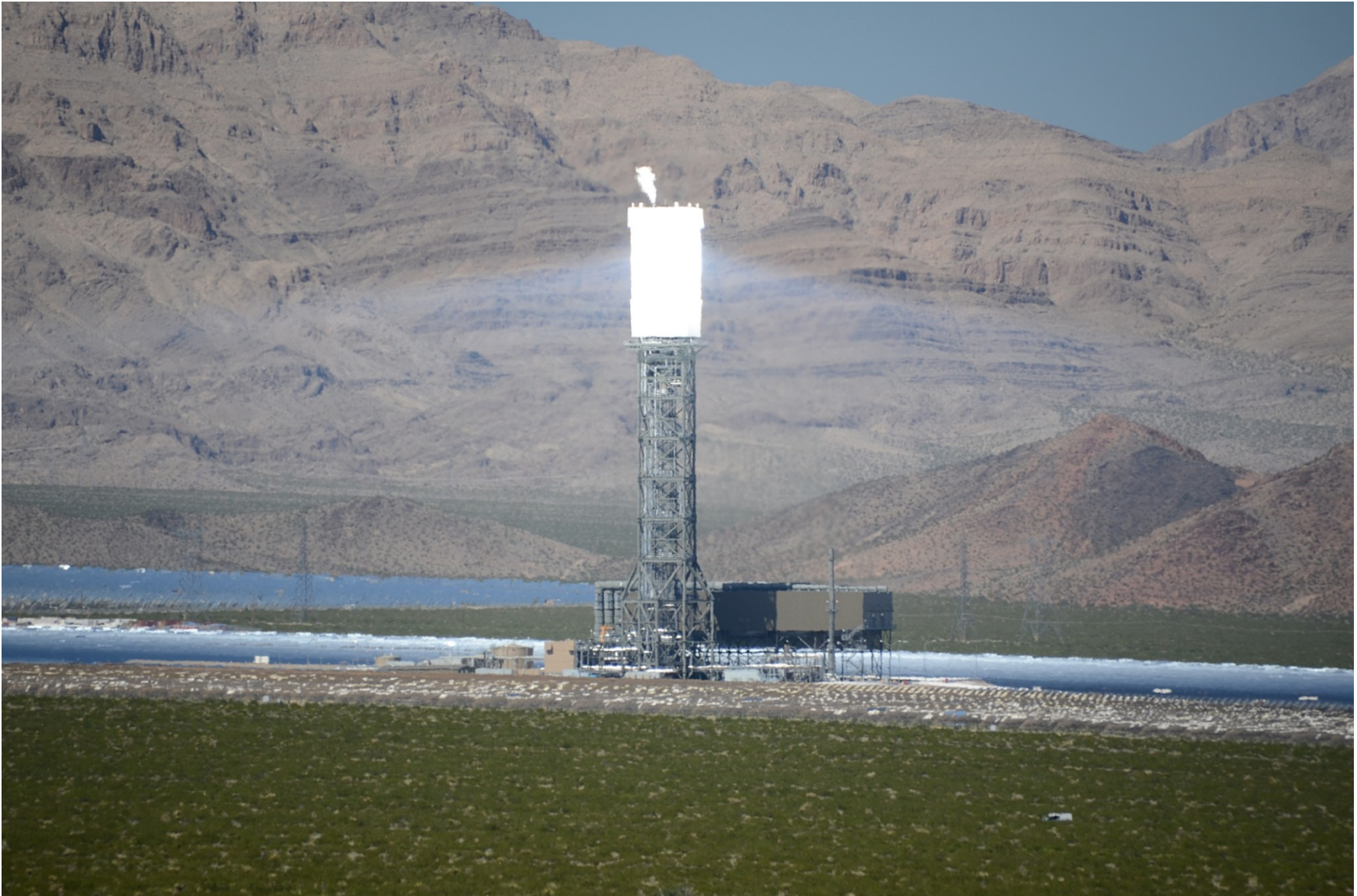
FIGURE 3.1-8 Fully Illuminated Receiver with No Surface Details Visible (Note small plume above receiver and dust halo.)
