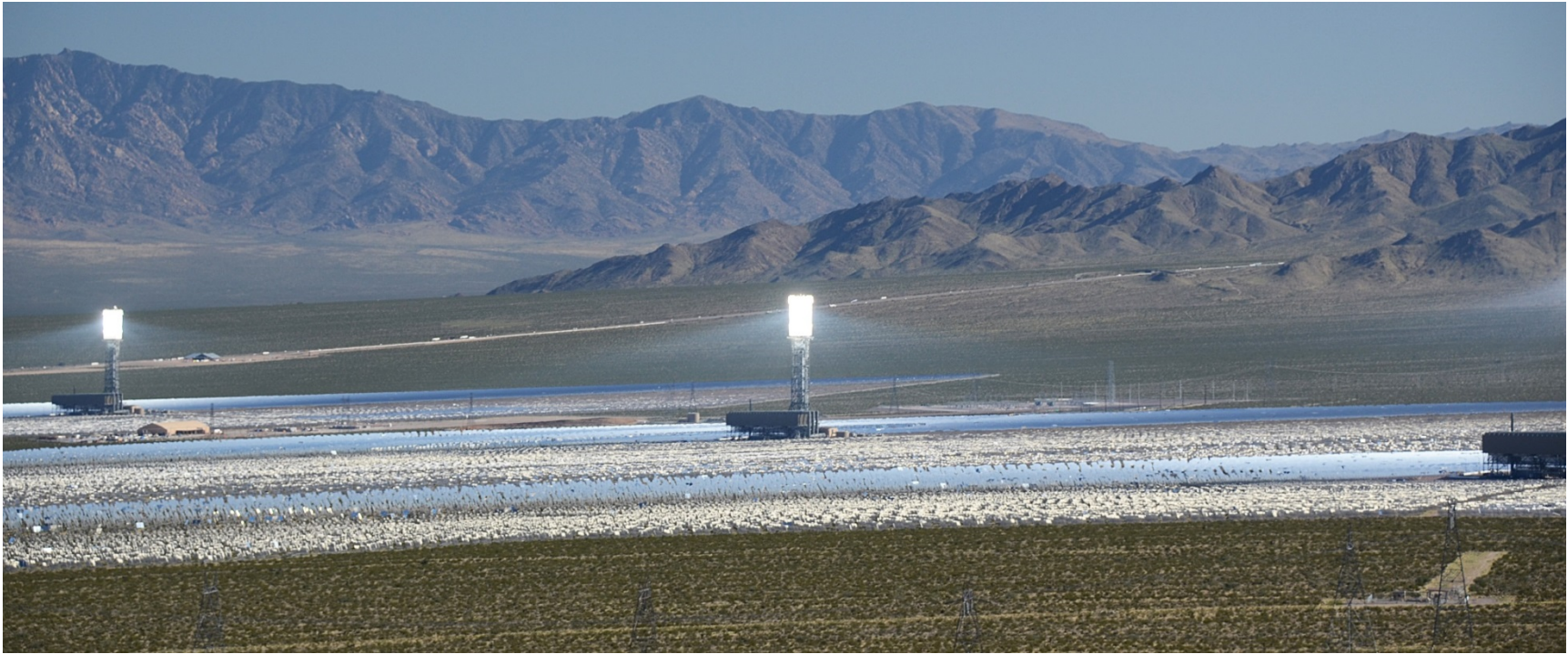
FIGURE 3.1-13 White Backs of Heliostats Visible on Heliostats Facing Away from the Observer. Photo location: SOP 13. Distance to Tower 2 is 4.3 mi (6.9 km). (Note prominent dust halos.)
