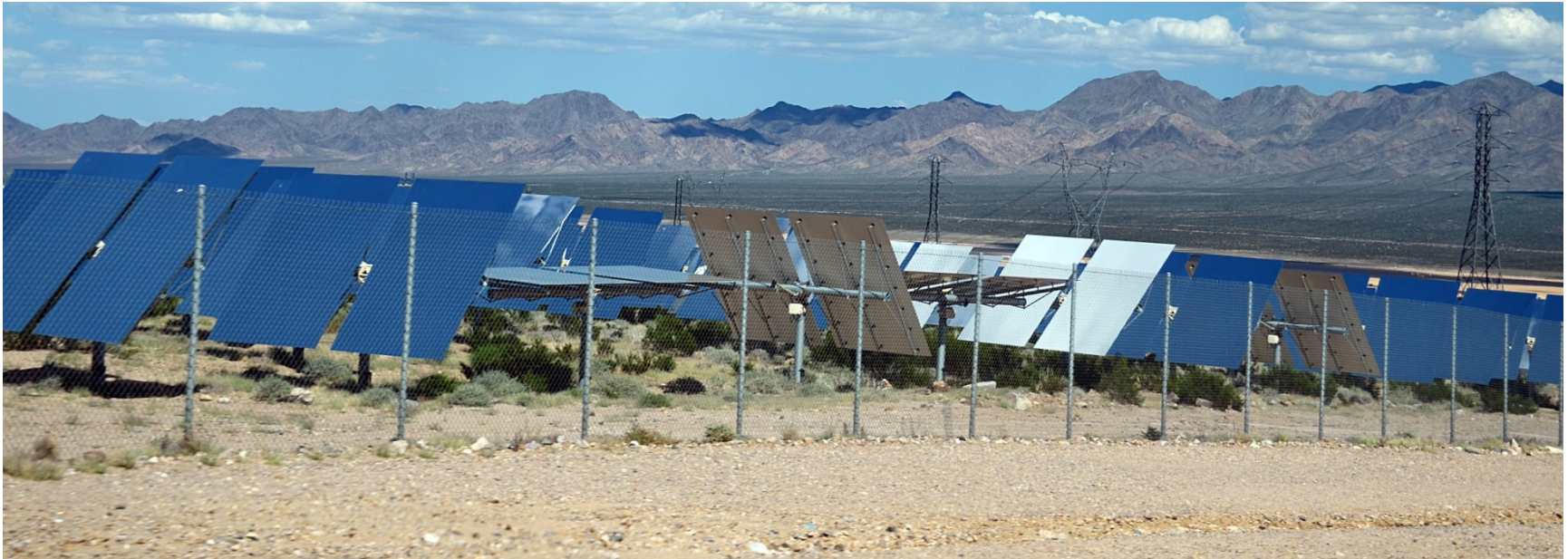
FIGURE 3.2-5 ISEGS Heliostats Pointed in Apparently Random Directions
