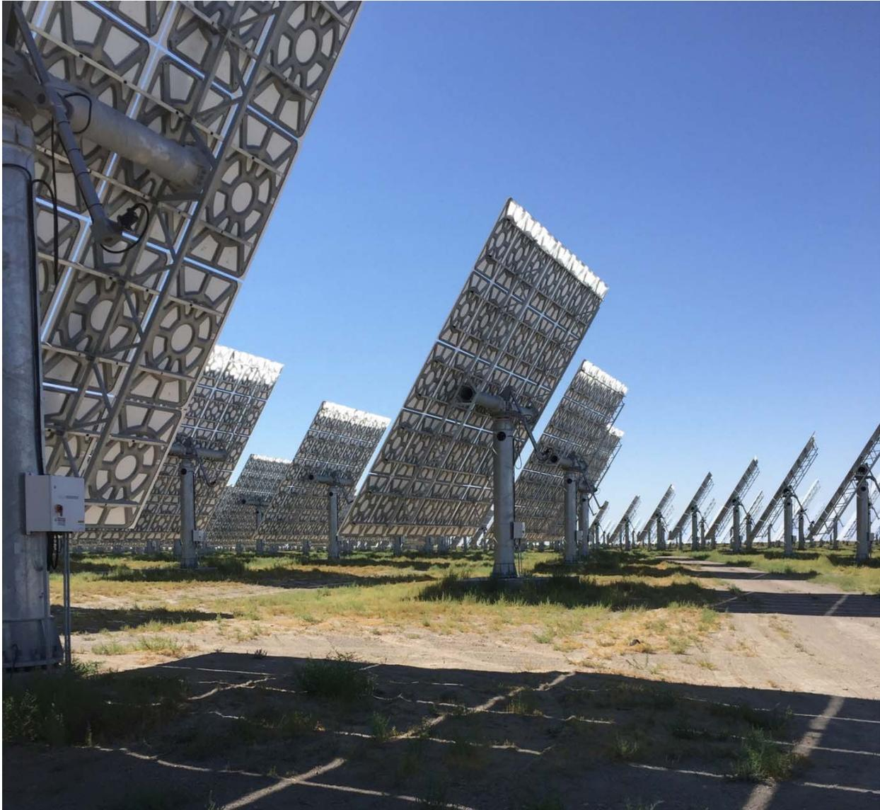
**FIGURE 5.3-8** Backs of Heliostats and Heliostat Support Structures Surrounded by Cleared Area
