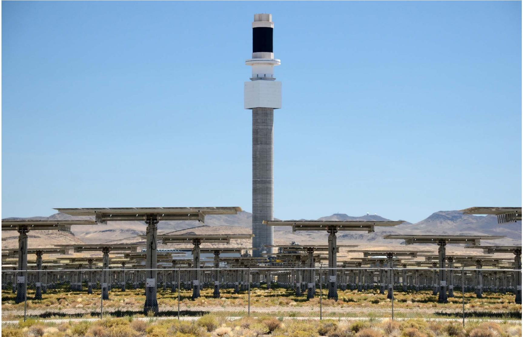
**FIGURE 3.1-4 CDSEF Offline. Receiver and Inner Portion of Heliostat Array with Heliostats in Stow Position.**
