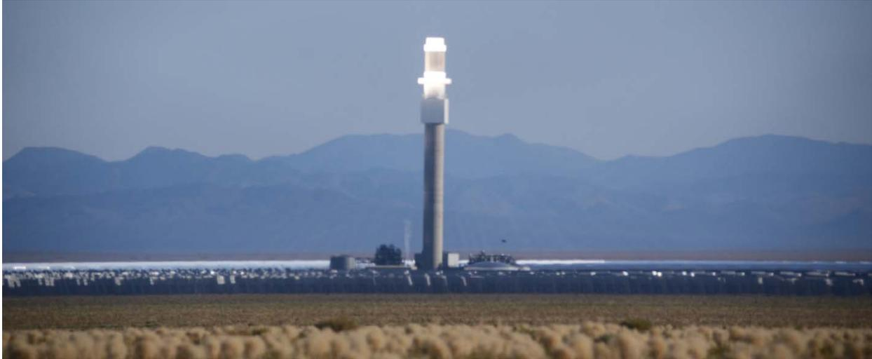
**FIGURE 3.1-7 Partially Illuminated Receiver, with Water Vapor Plume Immediately Left of Tower**
