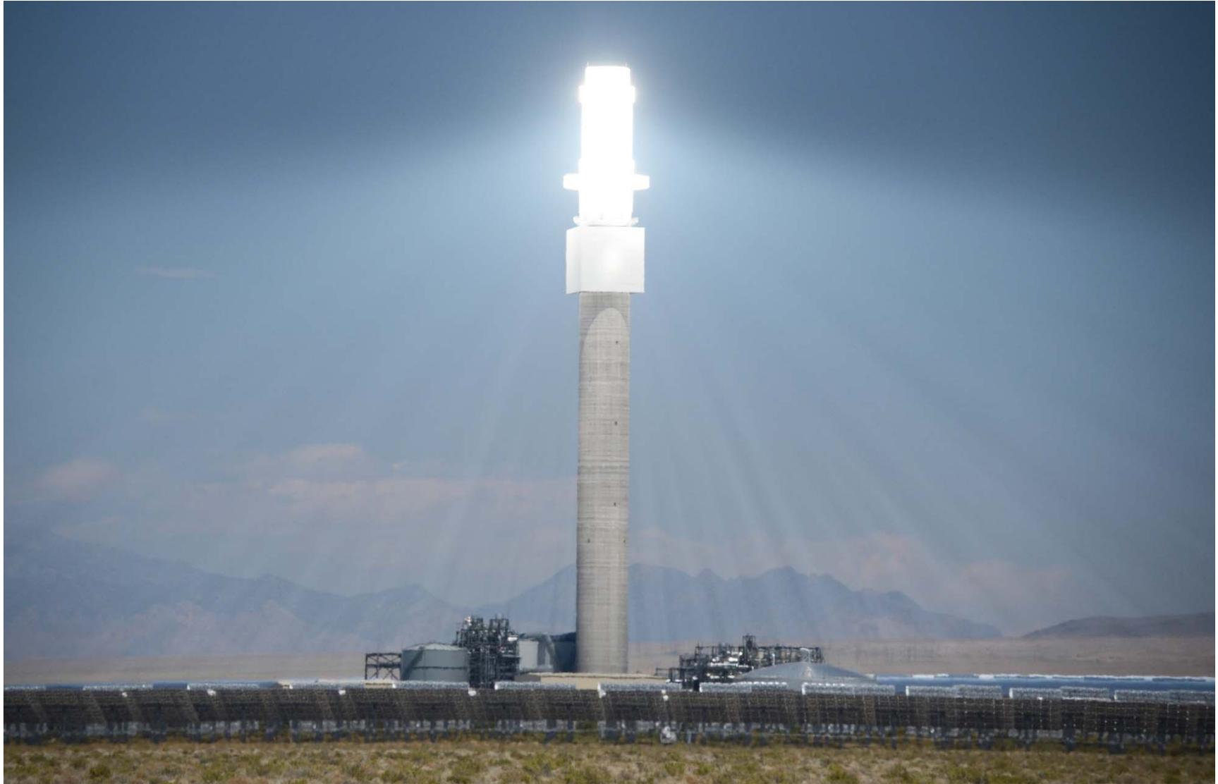
**FIGURE 3.1-3 CDSEF Operating Receiver, Power Block, and Inner Portion of Heliostat Array**
