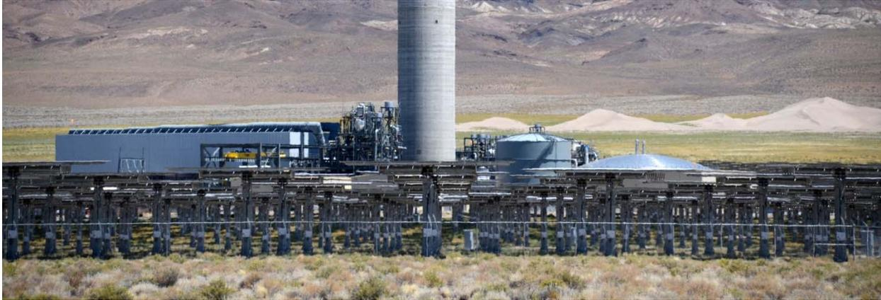
**FIGURE 3.1-10 Power Block Components. Air Cooled Condenser at Left, Top of Cold Salt Tank at Right. Steam Turbine/Generator behind Tower.**
