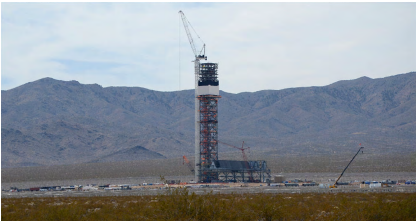
Ivanpah Solar Energy Generating System power tower under construction. The grayish area at center is a heliostat field for the central tower, one of three towers in the facility. The structure just to the right of the tower base will house the steam turbine generator. (Credit: Robert Sullivan, Argonne National Laboratory.)
