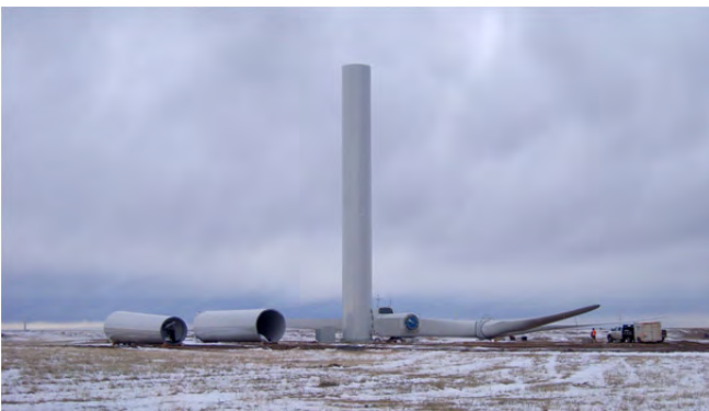
Partially erected turbine, with nacelle and hub visible at right center. (Near Peetz, Colorado. Credit: Robert Sullivan, Argonne National Laboratory.)
