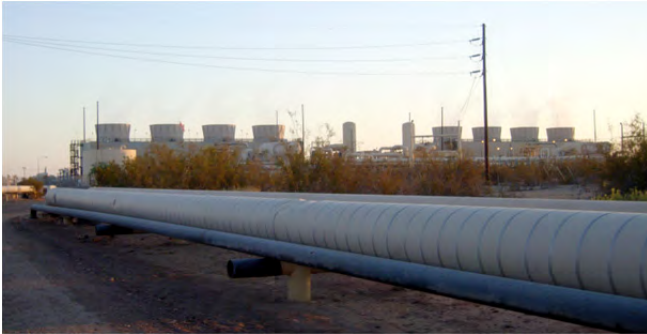
Pipelines and cooling towers at operating geothermal plant. (GEM 2/GEM 3 facility near Holtville, California. Credit: Robert Sullivan, Argonne National Laboratory.)
