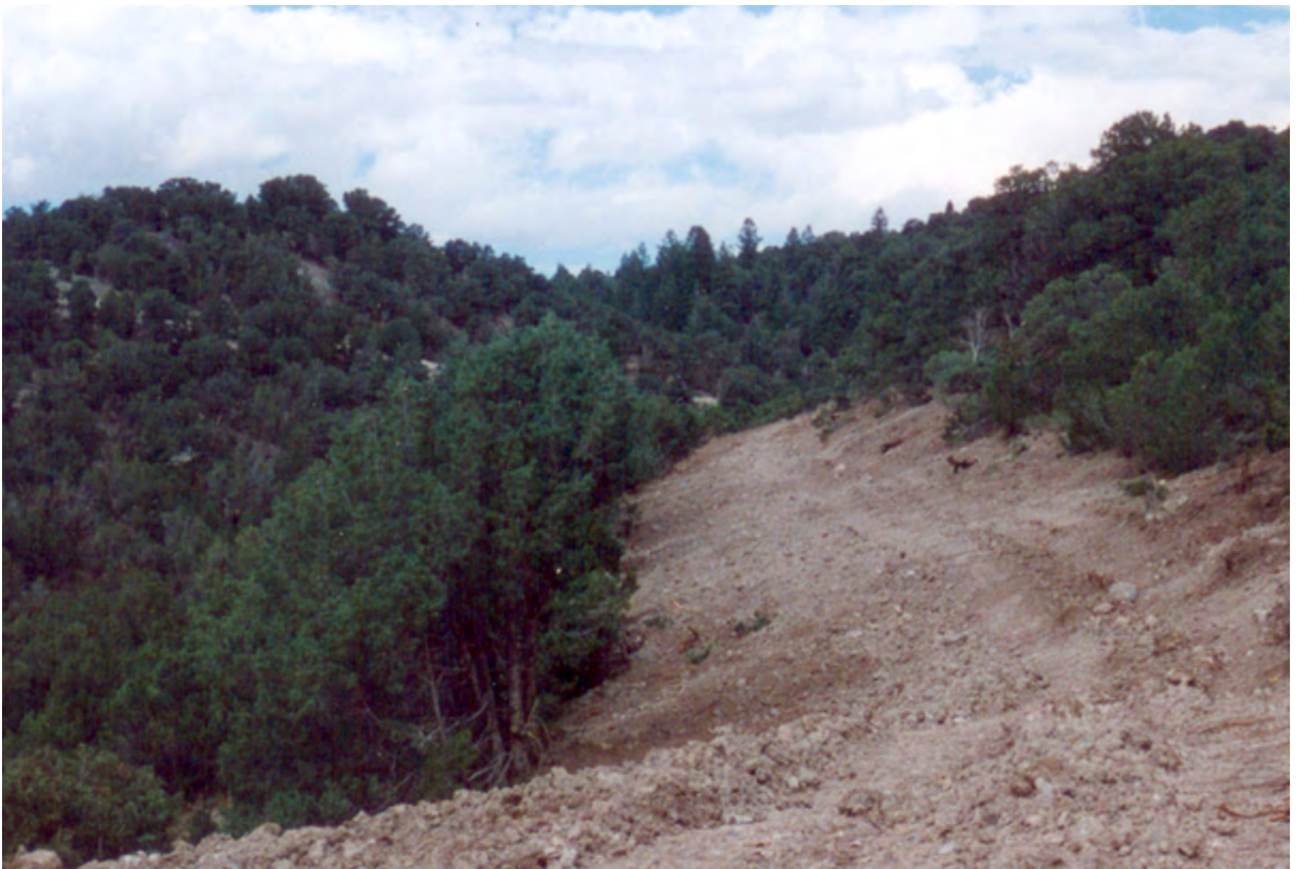
The recontoured slope for this reclaimed road blends in well with the naturally occurring slope. (Credit: BLM.)
