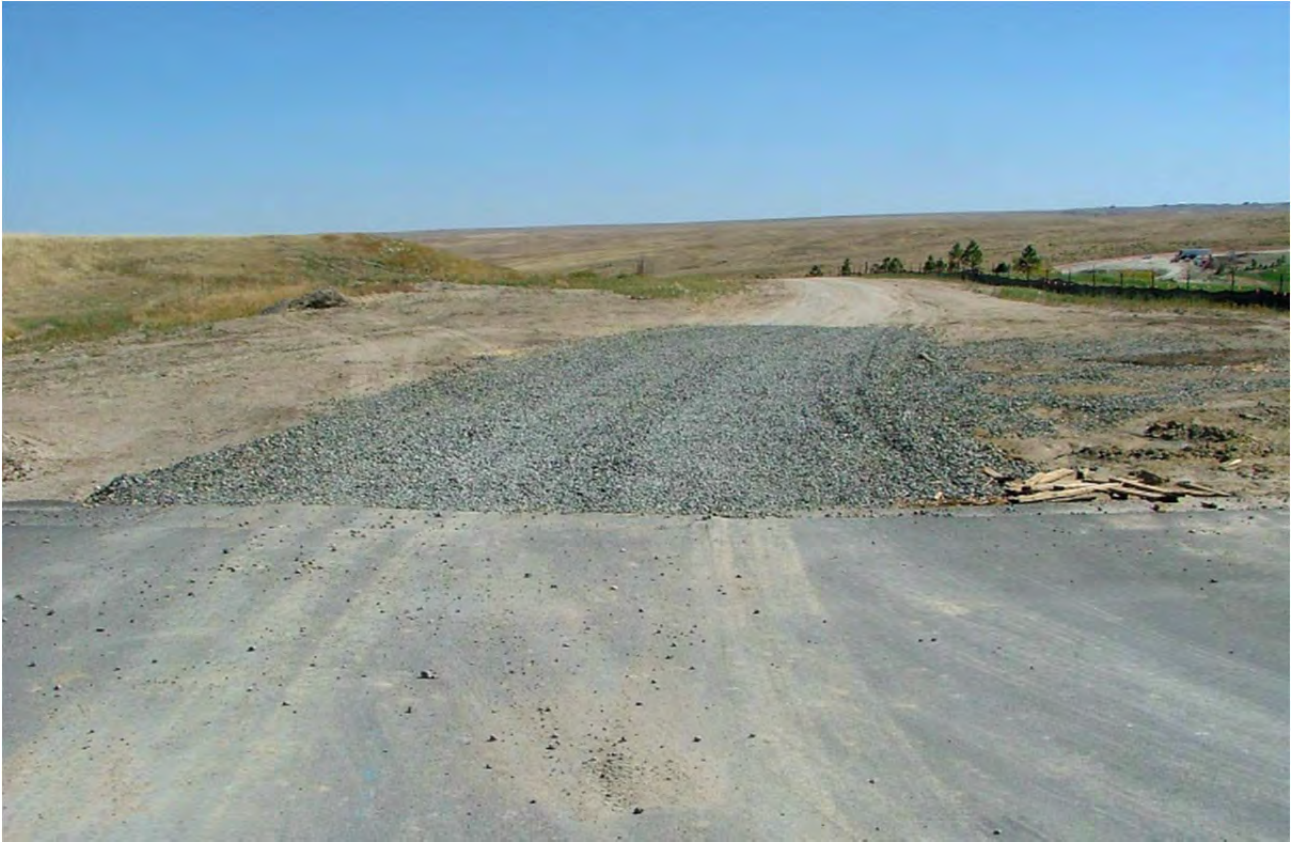
A vehicle tracking pad is typically a stabilized pad of coarse aggregate over a geotextile base installed at construction site exits to roadways. When vehicles drive over the pad, the tires sink into the rock slightly and mud on the tires is removed. (Credit: Tom Gore, Altitude Training.)
