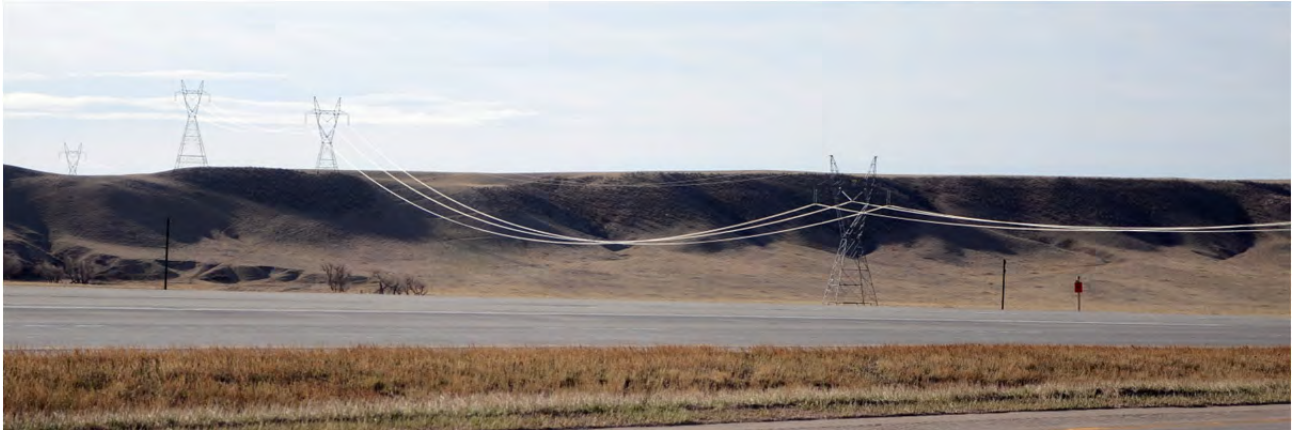
Failure to employ non-specular conductors for this transmission line result in high visual contrast in sunny conditions. (Credit: Robert Sullivan, Argonne National Laboratory.)
