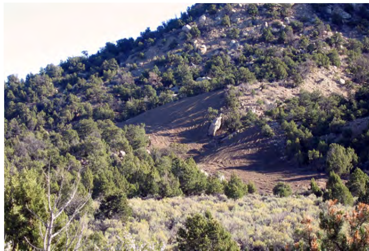
Burying a pipeline. Slopes are contoured to approximate naturally occurring slopes. (Credit: Rob Sweeten, BLM.)
