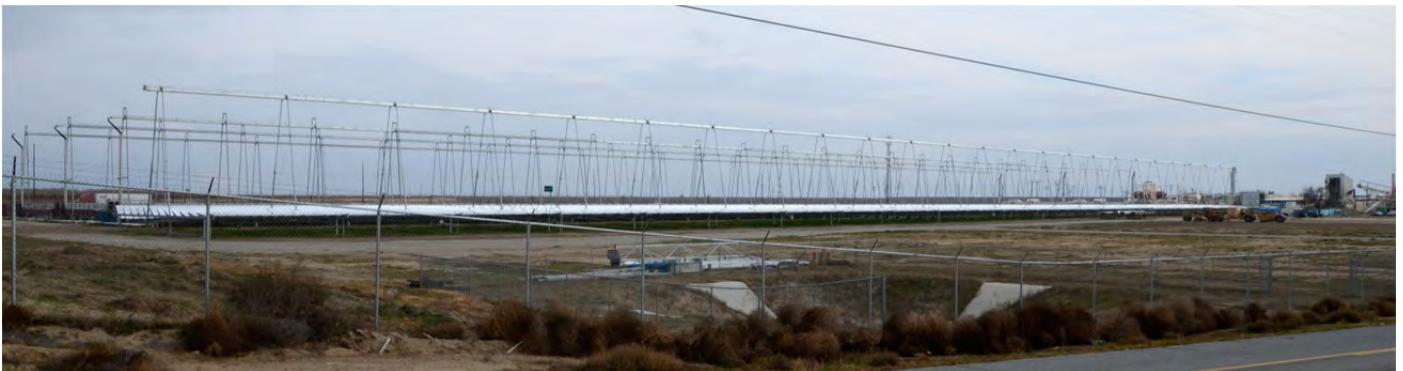
Close-up photo of Kimberlina CLFR facility near Bakersfield, California. Mirrors are the white band running left to right across the photo. The receiver tubes are held well above the mirrors. Ancillary buildings, including STG, are at far right. (Credit: Robert Sullivan, Argonne National Laboratory.)
