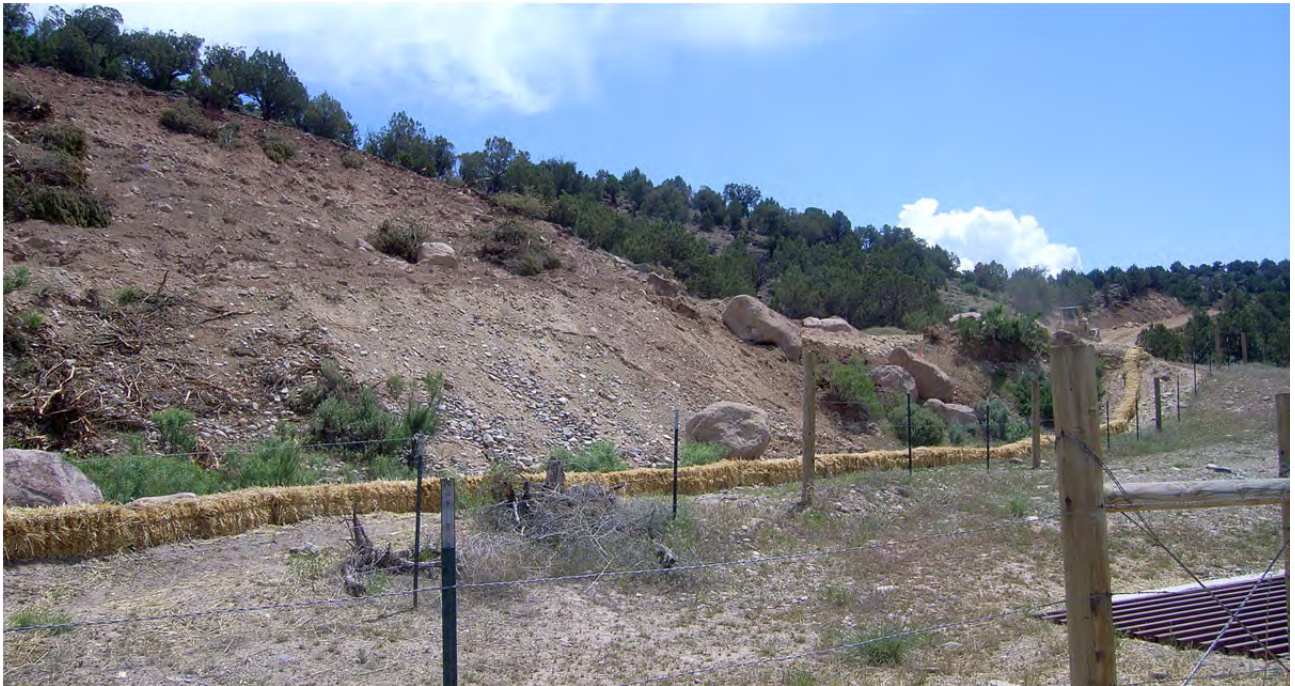
An example of erosion control good practices: straw bales used for downslope sediment control. (Credit: BLM.)
