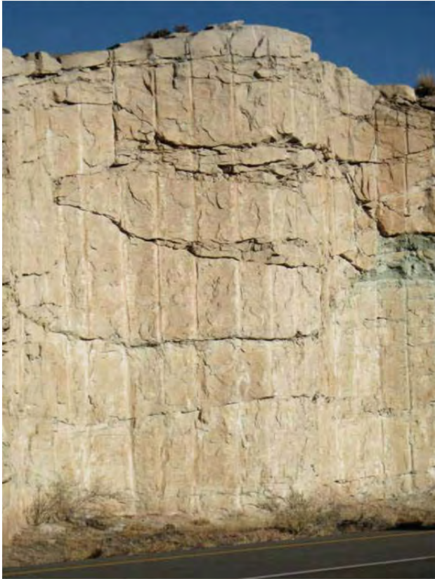
Half cast drill traces in sandstone have an obvious artificial appearance. (Credit: U.S. Department of Transportation Federal Highway Administration.)
