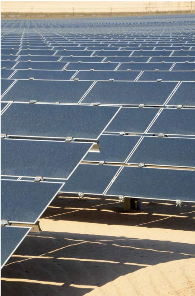
Flat plate PV: Thin-film PV panels on fixed (non-tracking) mounts. (Silver State North Solar Project near Primm, Nevada. Credit: Robert Sullivan, Argonne National Laboratory.)
