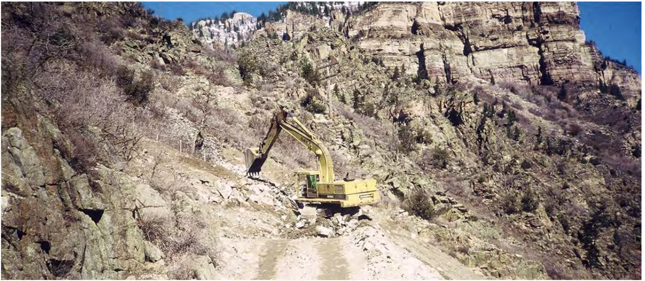
Slope recontouring for road reclamation. (Credit: John McCarty, Colorado Department of Transportation.)
