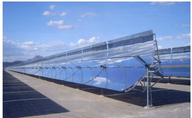
Parabolic trough assembly at a parabolic trough facility, including large curved reflectors, the HTF tube at the focal point of the reflectors, and the support structure behind and below the reflectors. (Nevada Solar One near Boulder City, Nevada. Credit: Robert Sullivan, Argonne National Laboratory.)
