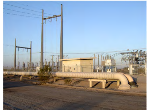
Geothermal pipelines coated to match surroundings at dual-flash geothermal power plant. Note that better results would have been obtained by using a darker color shade on the pipe coating. (GEM 2/GEM 3 facility near Holtville, California. Credit: Robert Sullivan, Argonne National Laboratory.)
