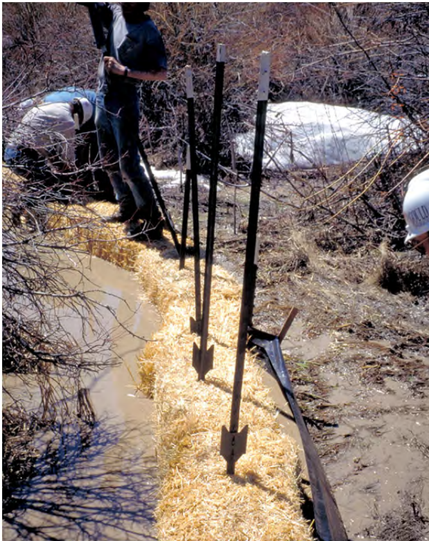
Although imperfectly installed, this combination of straw bales and silt fence is holding back a large amount of water and sediment. (Credit: John McCarty, BLM.)
