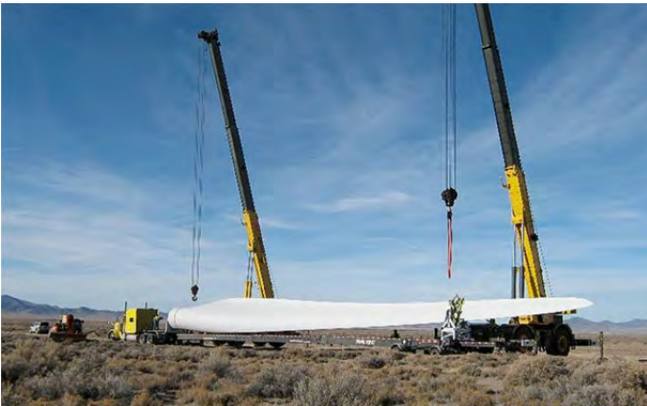
Unloading a wind turbine blade. (Milford Wind Corridor project, near Milford, Utah. Credit: BLM.)
