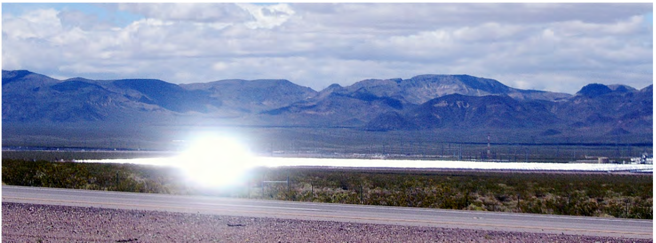
Offsite glare from parabolic trough facility as seen from highway, approximately 1.9 mi from glare spot. (Nevada Solar One facility near Boulder City, Nevada. Credit: Robert Sullivan, Argonne National Laboratory.)
