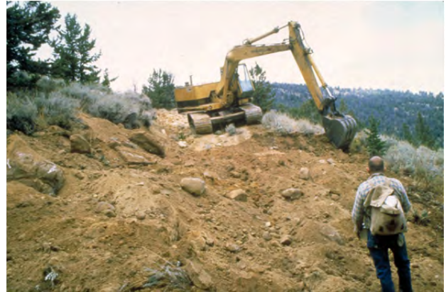
Slope recontouring to approximate naturally occurring slopes during road reclamation. (Credit: BLM.)
