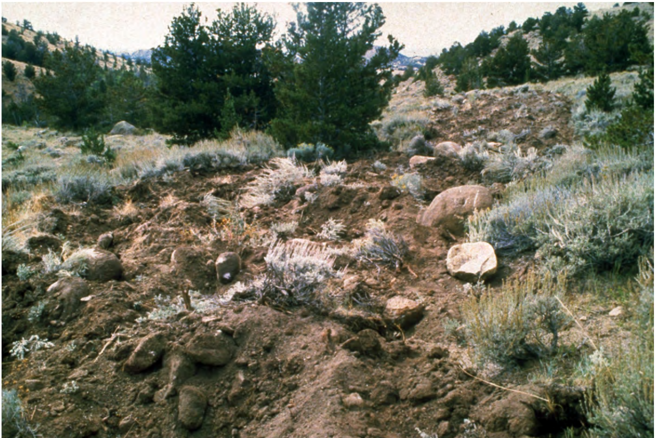
Road removal in progress. The flat road surface is roughened, rocks are added, and vegetation transplanted from the edges of the ROW. (Credit: BLM.)
