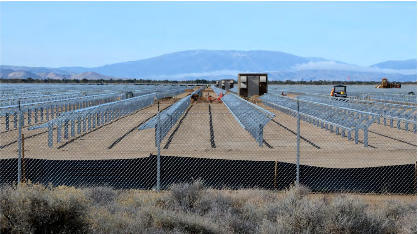
Antelope Valley Solar Ranch thin-film PV facility under construction. Fixed (non-tracking) mounts for the PV panels have been installed, and await the panels. Note complete clearing of vegetation and leveling of ground underneath the collectors. (Credit: Robert Sullivan, Argonne National Laboratory.)
