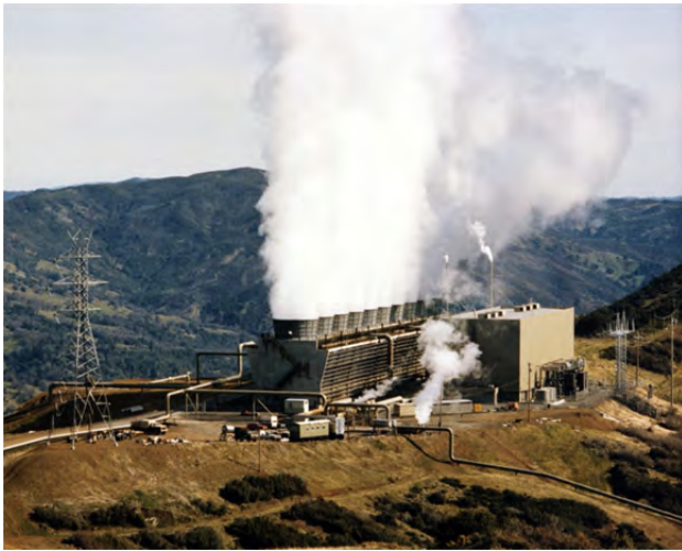
Steam plumes rise from cooling towers at a dry steam plant. (Geysers facility near Calistoga, California. Credit: NREL.)
