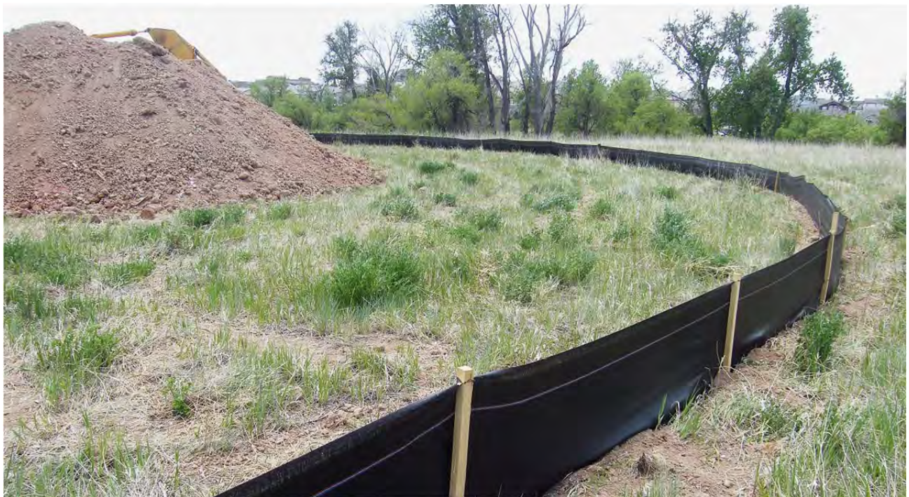
Stockpiled topsoil, surrounded by a silt fence intended to control offsite soil transport during heavy rains. (Credit: BLM.)
