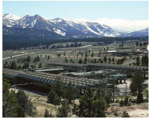
Air-cooled geothermal plant. The use of dry cooling technology avoids visual impacts from plumes. Note the use of vegetation for partial screening of ground-level views of the plant. (Mammoth facility, eastern Sierra Nevada in California. Credit: NREL.)
