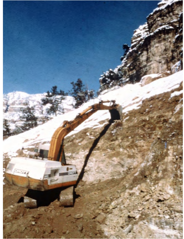
Proper replacement of this rock shelf preserves the form, line, and texture of the original rock shelf, and color contrast will be greatly reduced when revegetation occurs. (Credit: John McCarty, Colorado Department of Transportation.)
