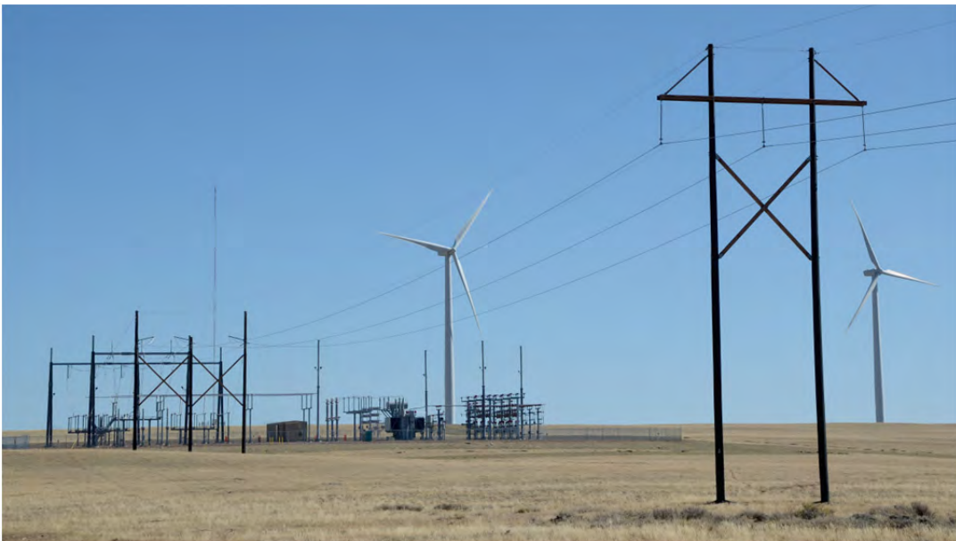
Wind energy facility substation, with meteorological tower in background. (Dunlap Ranch Wind Energy Project near Medicine Bow, Wyoming. Credit: Robert Sullivan, Argonne National Laboratory.)
