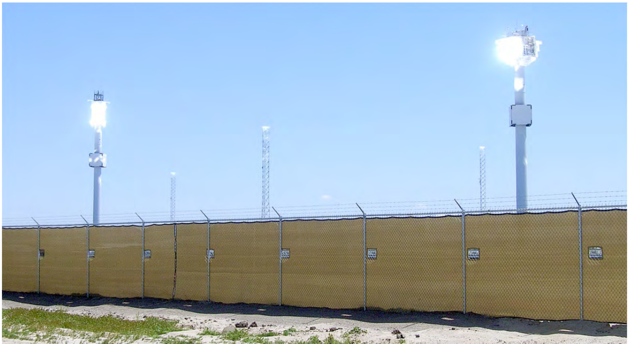
A fabric-covered screening fence at power tower facility screens the heliostats, but not the receivers. (eSolar Sierra Suntower, Lancaster, California. Credit: Robert Sullivan, Argonne National Laboratory.)
