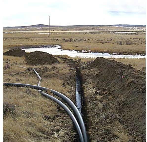
Burying a small pipeline. (Credit: BLM.)
