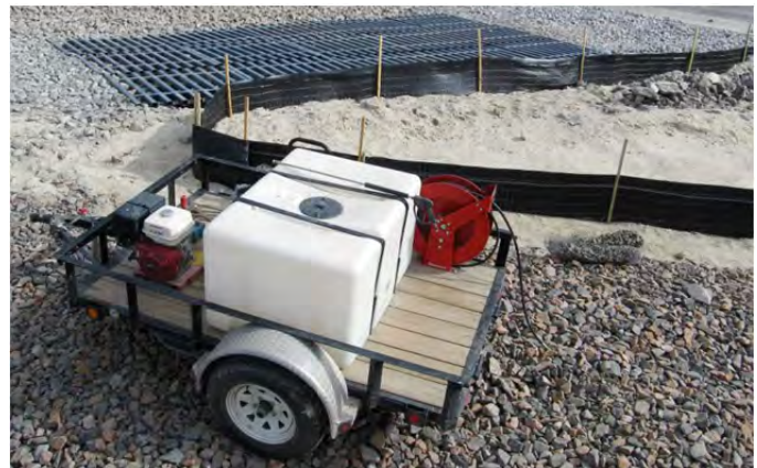
An exit tire wash removes dust, soil, mud, and other materials from trucks to minimize potential trackout of material onto roadways. (Credit: Tom Gore, Altitude Training.)
