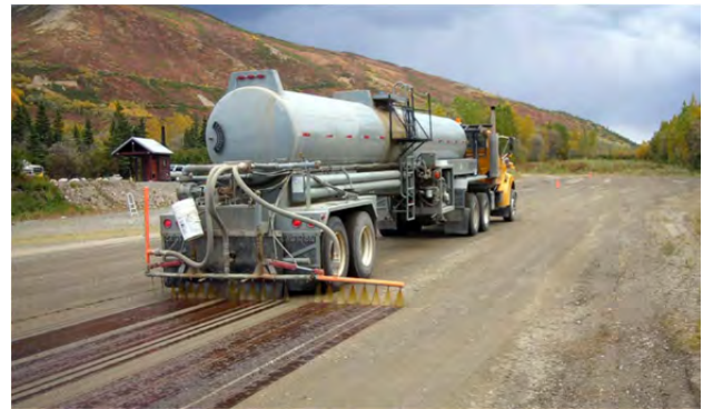
Application of dust palliative. (Credit: Alaska Department of Environmental Conservation, Division of Air Quality.)
