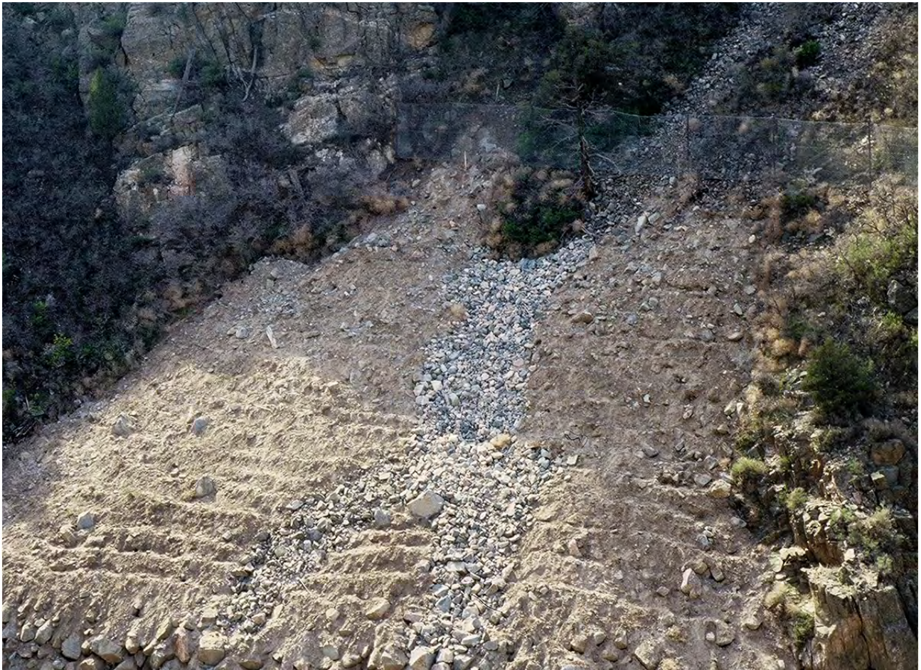
Furrowing slopes results in increased water retention, reduced erosion, and better revegetation. (Credit: John McCarty, Colorado Department of Transportation.)
