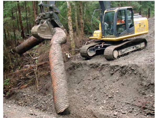
Culvert removal during road decommissioning. (Credit: Washington State Recreation and Conservation Office.)
